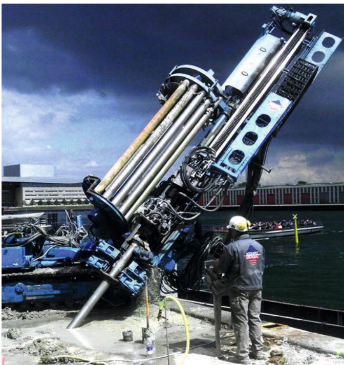
Image 1: Our drill rig drilling „over head“
