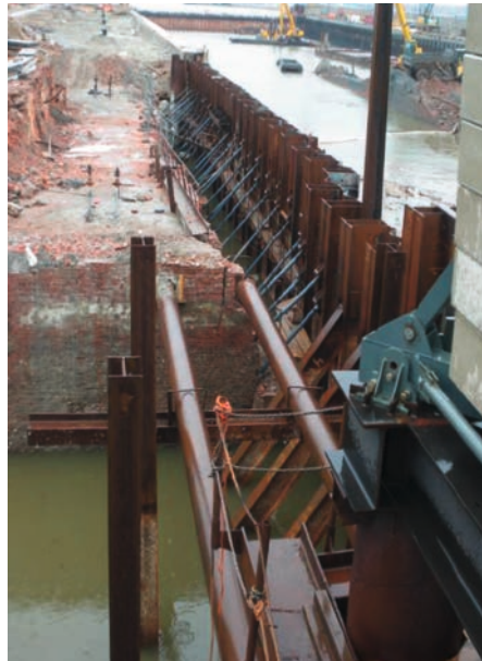
Images 8a and 8b: side cut of chamber wall west near the former outer lock head and side view of the finished micropiles lining the chamber wall.
