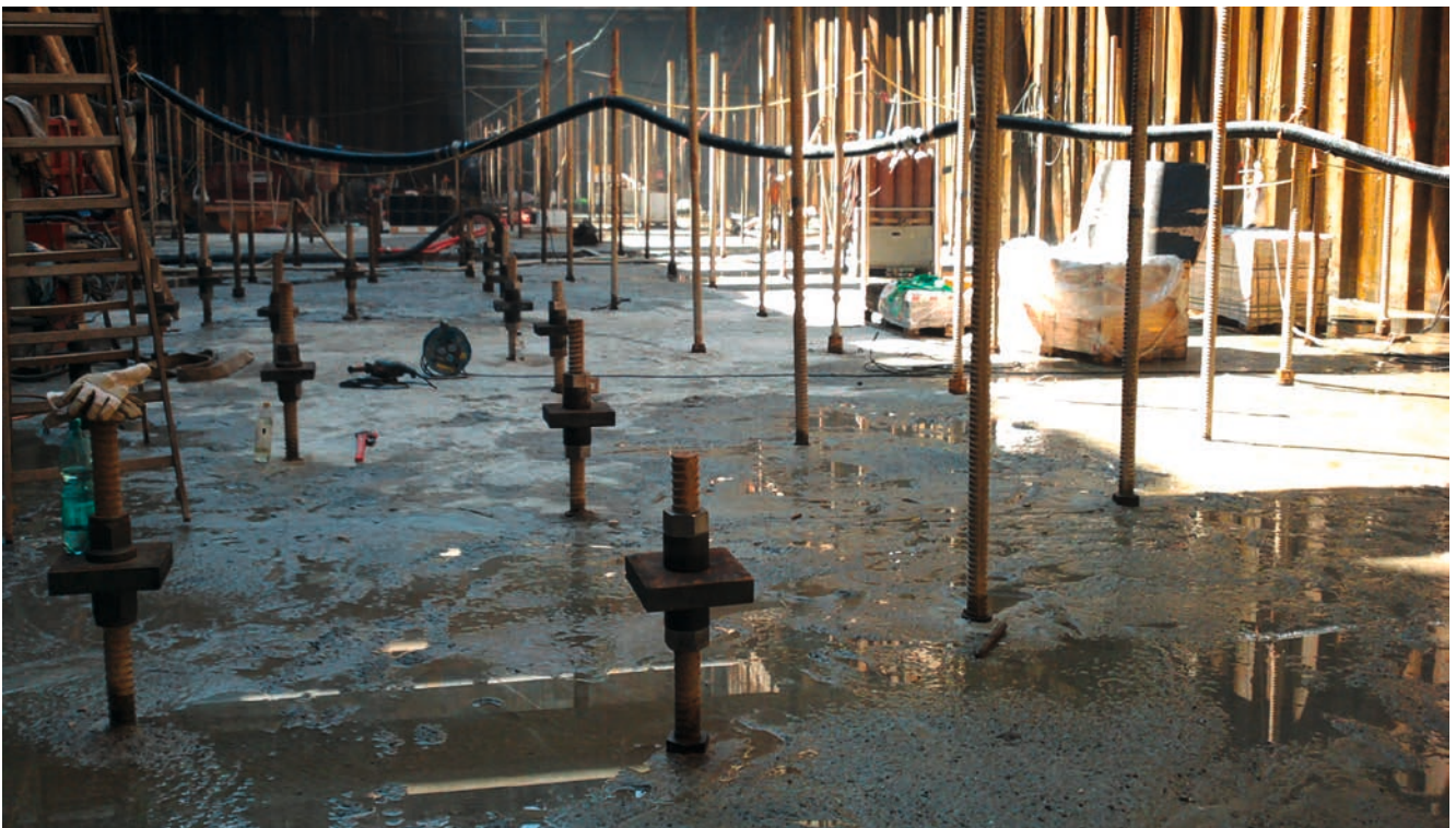
Image 6: view onto the finished pile heads in the dewatered gate chamber
