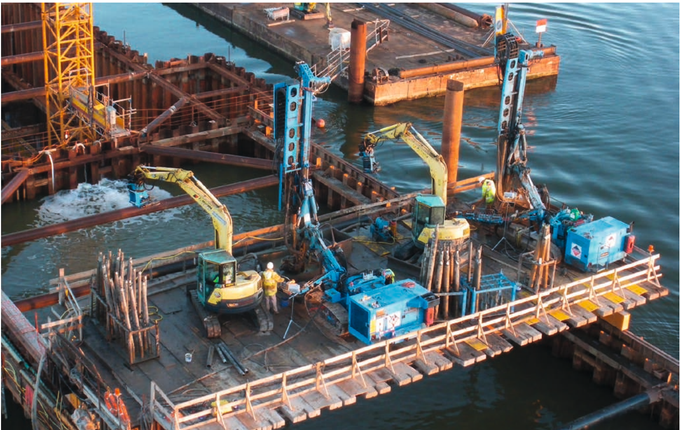
Image 4: View onto the mobile work platform near the gate chambers
