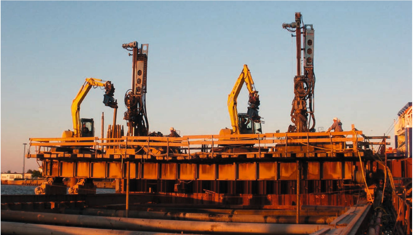
Image 5: view onto the mobile platform with two drill units near the gate chambers
