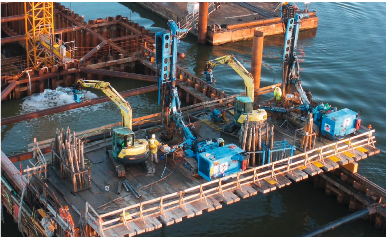
Image 7: Work unit on top of a stilted platform at the chamber wall west
