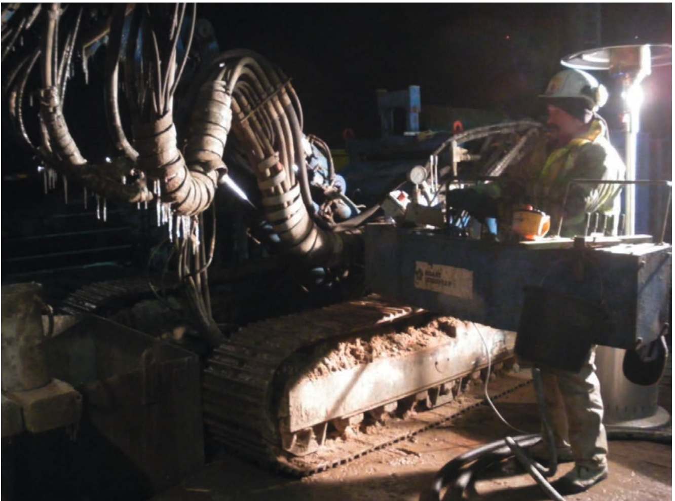
Image 11: drill works under extreme weather conditions at night in January 2010
